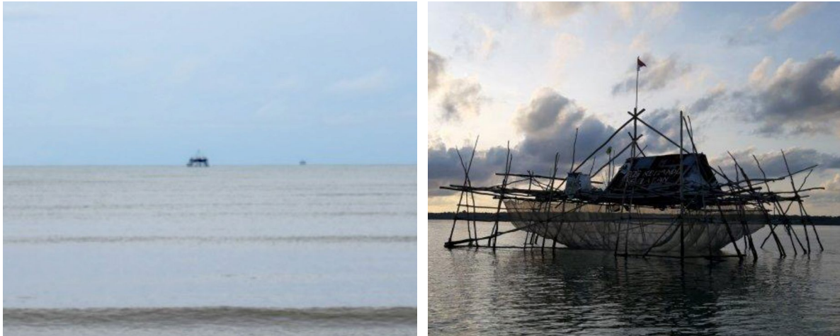
Figure 31. Bagan in Tanah Kuning (Left), Closer View (Right).
